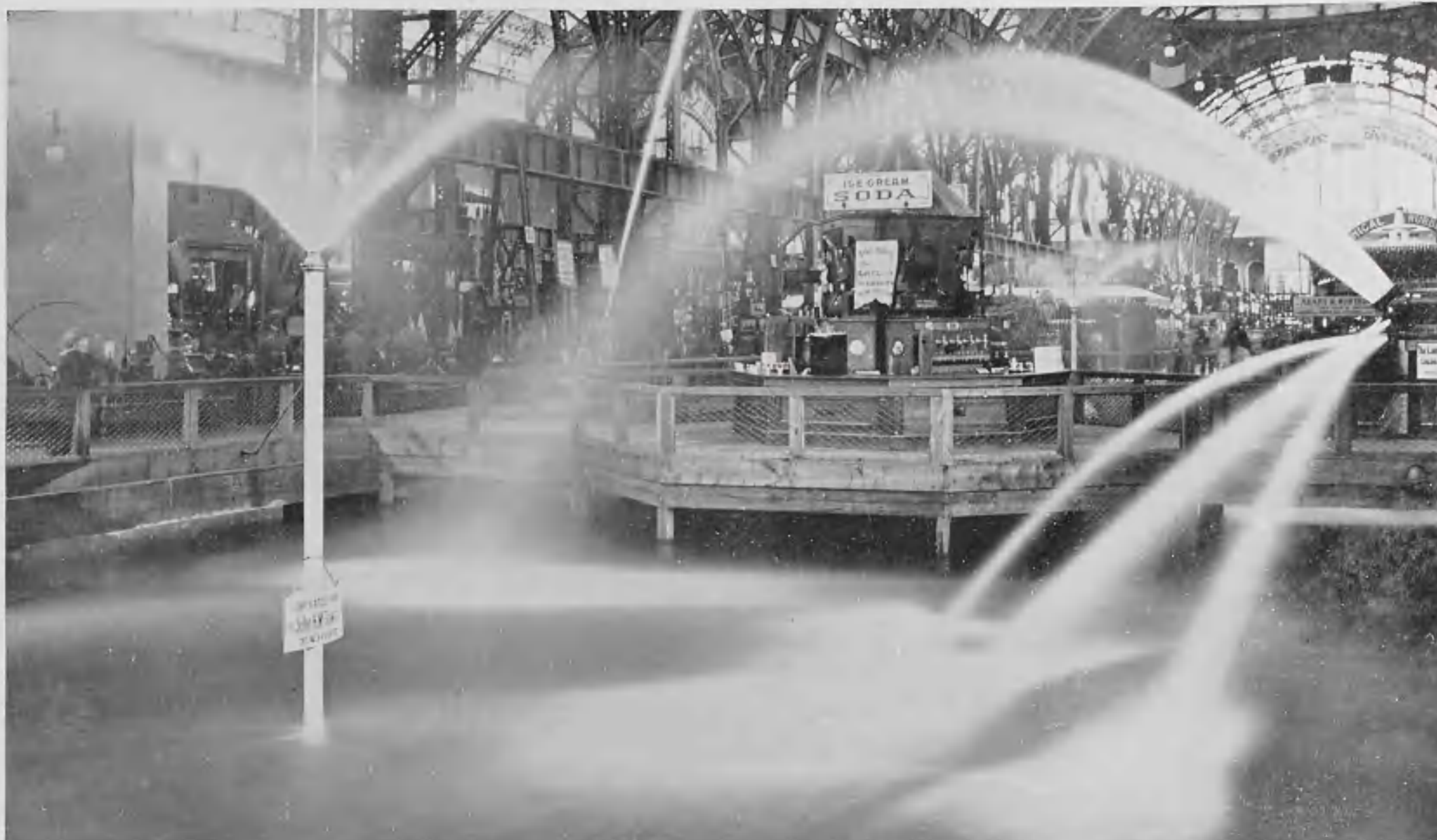
FOUNTAINS, PUMPING ENGINE EXHIBIT
